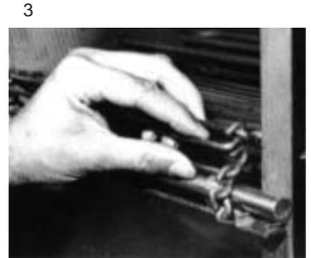
To reassemble, reverse the procedure. Be sure to reassemble the belt with the knuckle opening facing away from the direction of travel.
