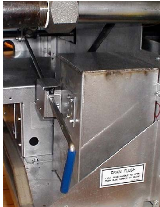
Drain-flush handle (blue) location.
